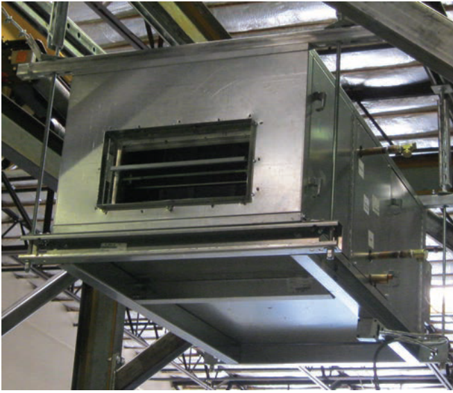
FIGURE 2 - SECTIONS OF STRUT ARE USED TO HANG THE UNIT
