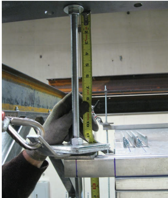
FIGURE 4 - RECOMMENDED LENGTH OF THREADED ROD
