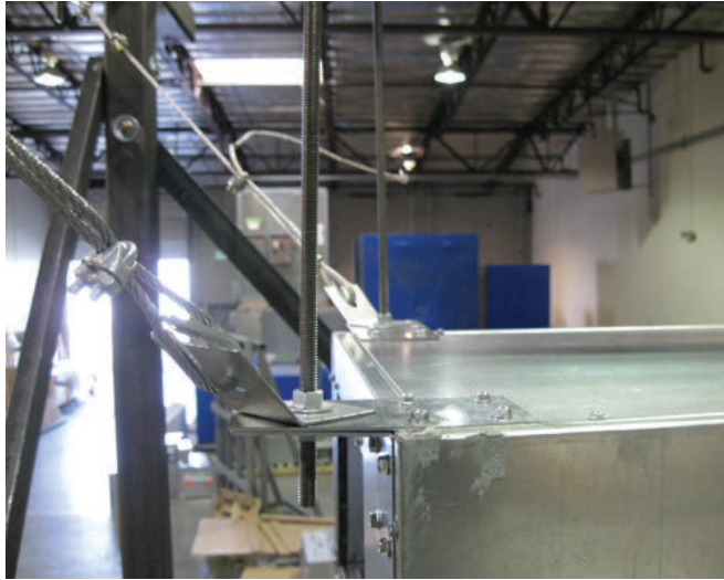
FIGURE 5 - OVERLAPPED FLAT, 90° AND 45° BRACKETS
