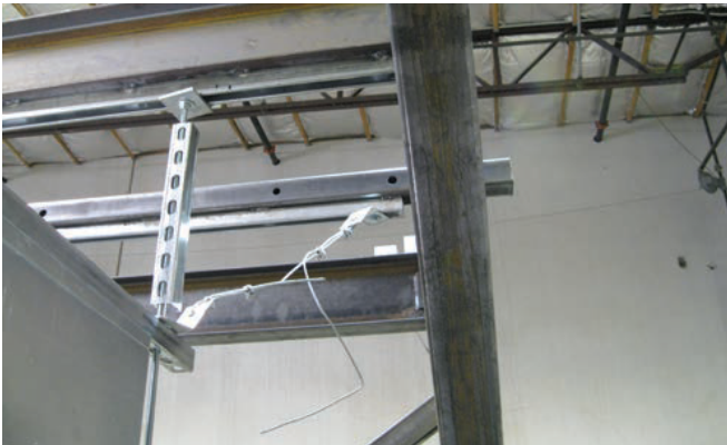
FIGURE 3 - LATERAL SUPPORT COMPONENTS FOR TBHD 08-20
