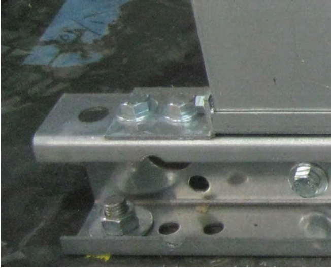
FIGURE. 10 - BOLT AT EACH BASE-RAIL CORNER
