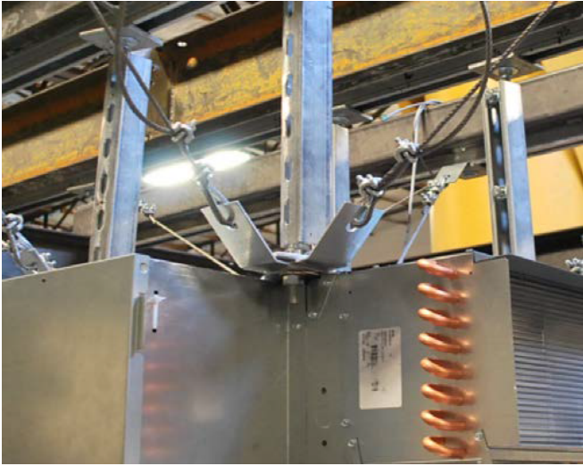
FIGURE 7 - OVERLAPPED FLAT AND 45° BRACKETS
